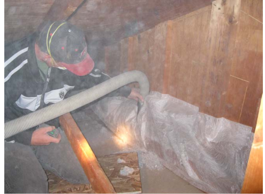
Blowing in new insulation
