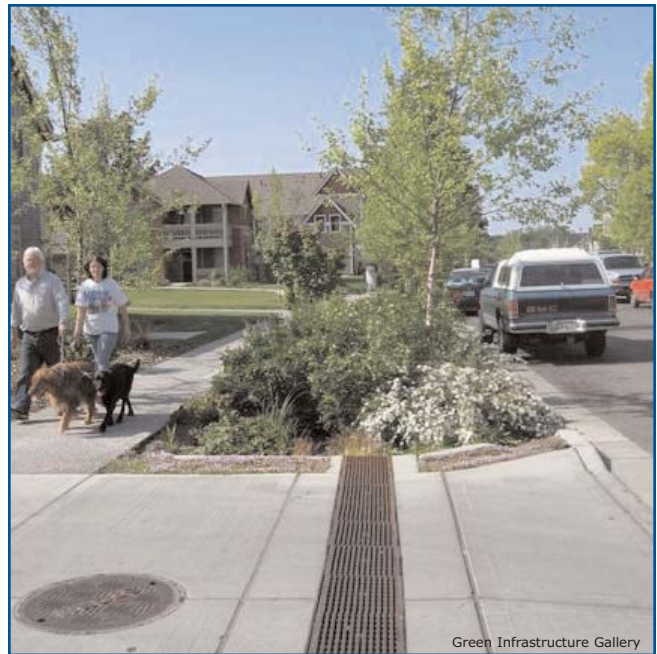
This catchment drain illustrates how to render a site's impervious cover "ineffective." The drain intercepts water that would otherwise flow into the street, directing flow into planters.
