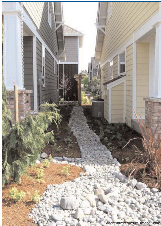
Small spaces between housing can be used for stormwater management. Note that codes limiting use of non-plant material would prohibit this BMP design.
