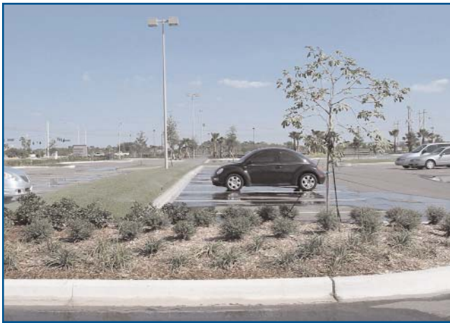
Code language directing islands and irrigation, combined with poor practices, creates runoff during dry weather.
