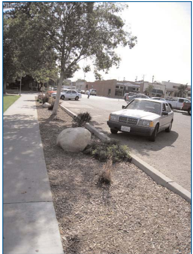
Requirements for continuous elevated curbs surrounding landscaping in parking areas prevents the use of such areas for drainage. Small curb cuts or other designs can allow runoff to enter landscaped areas to slow and filter runoff.
