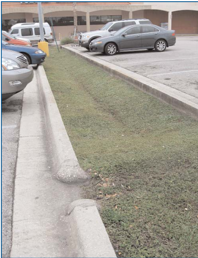
This mall is slated for redevelopment. In the short term, elevated beds were dug out and inlets constructed.
