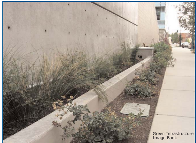
These planters in Emeryville, CA, are designed with overflow boxes and underdrains.
