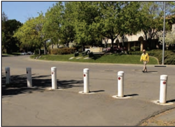
Posts with “knock down” capability for emergencies.
