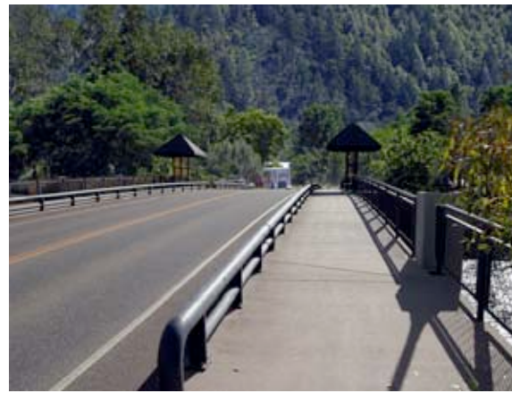
Trinity River Bridge—After
