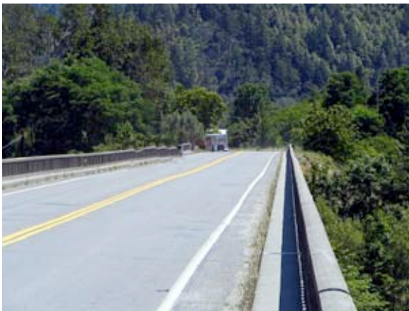
Trinity River Bridge—Before
