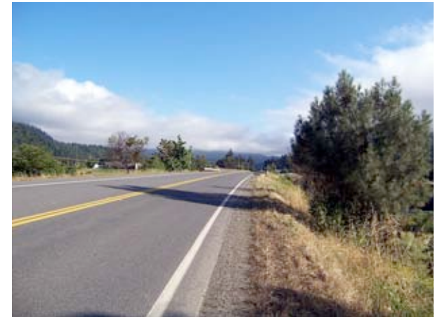
Highway 96 approaches the Trinity River Bridge northbound.
