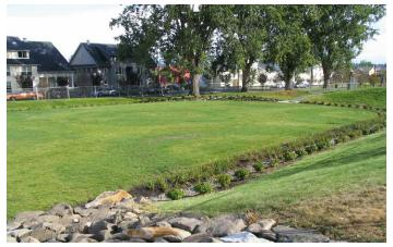
Figure 5–13 Project Precedent - Linear Vegetated Swale Encircling a Park
