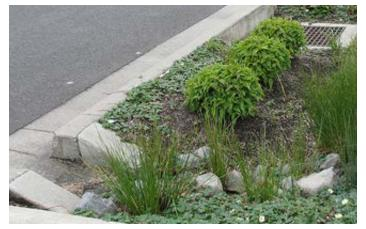
Figure 5–14 Project Precedent - Vegetated Swale with Concrete Inlet to Capture Drainage from Adjacent Roads
