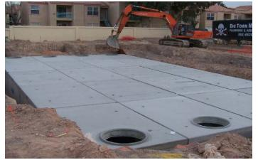
Figure 5–23 Project Precedent - Underground Infiltration Gallery with Access Ports (Las Vegas, NV)
