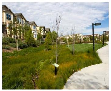
Figure 5–9 Project Precedent - Linear Bioretention in Mixed-use Development (Ladera Ranch, CA)
