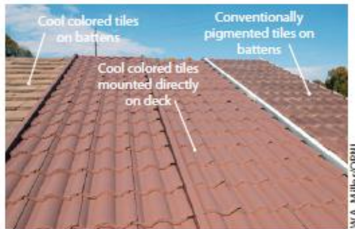
Figure 2. Conventional and Cool Colored Tiles (EPA 2011)
