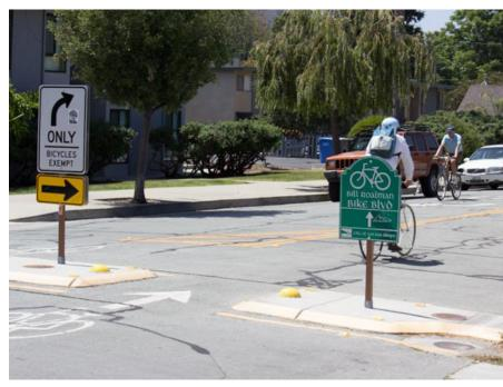
FIGURE 45: TRAFFIC CALMING DIVERTER - BIKE BOULEVARDS
