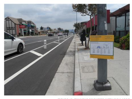
FIGURE 40: EXAMPLE OF BUFFER WITH BOLLARDS
