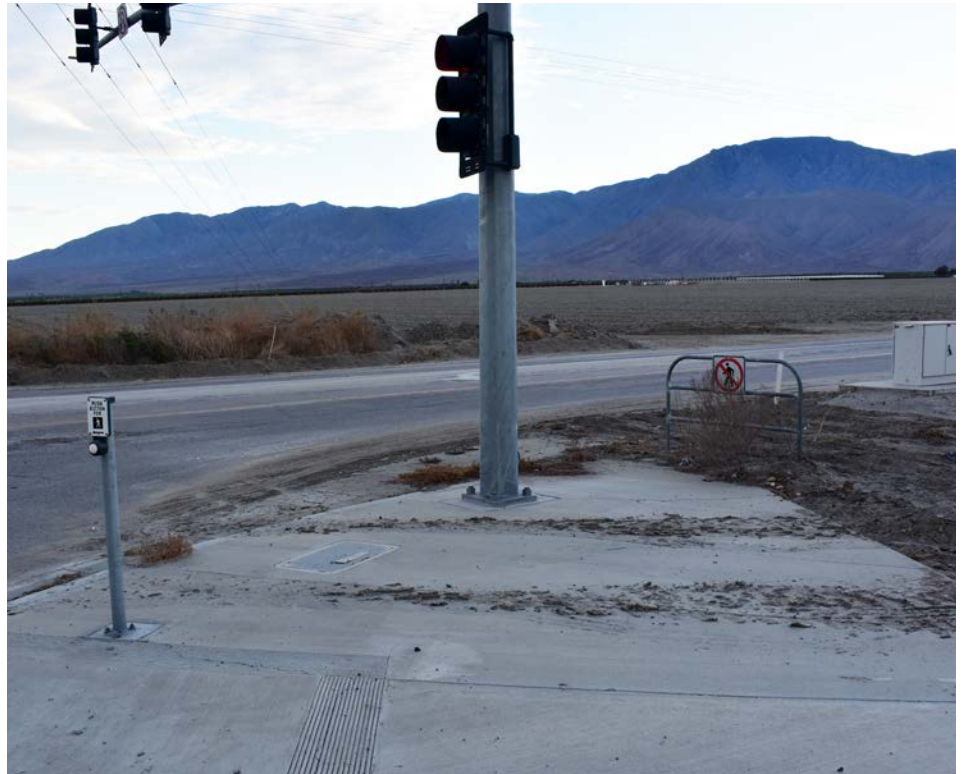
Signalized intersections have no connection to further pedestrian facilities
