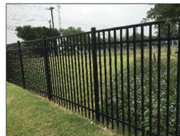
3 FOOT HIGH TUBULAR STEEL FENCING
